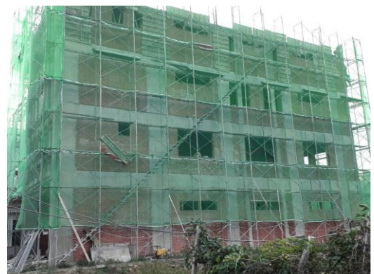
The new San Wan Church building project.
